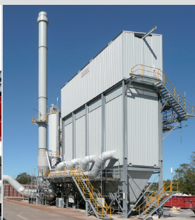
HKD-R - Hose filter plant HKD-R - Schlauchfilteranlage
